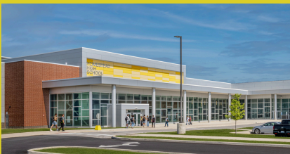
Homestead High School Expansion & Renovation
